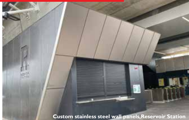
Custom stainless steel wall panels, Reservoir Station
